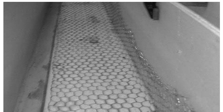
Figure 6: The flood plain wall which is clench in place
