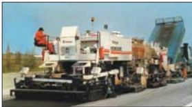
Figure 3: Hot In-Place Recycling [4]
