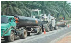
Figure 5 Typical Cold In-Place Recycling Train
