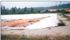
A lined cell in a landfill to prevent contamination from leachate generated in the cell
