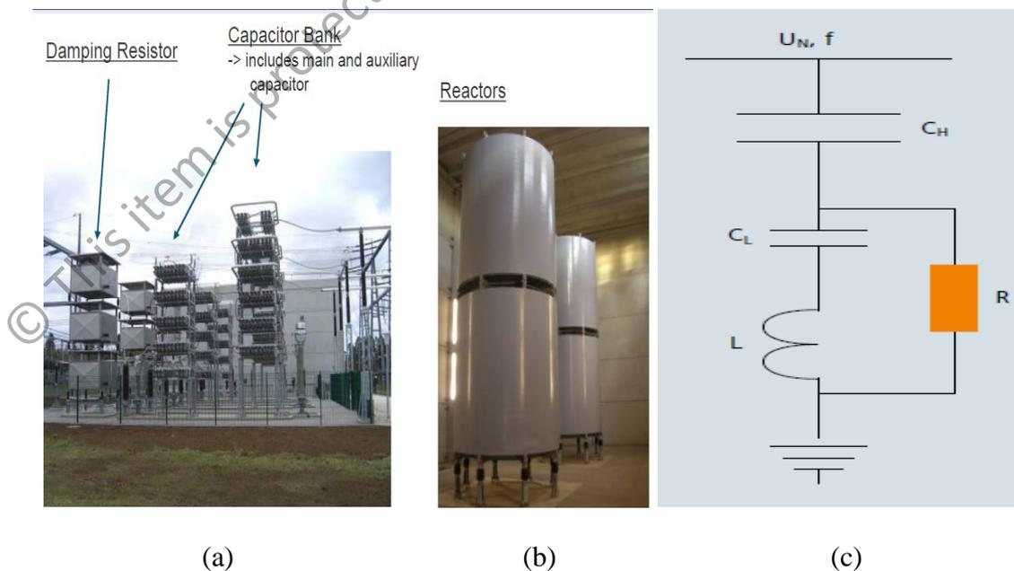
Figure 1.1: (a) Real MSCDN (b) Real filter reactors (c) Simplified single line of MSCDN (Kampa, 2012).
