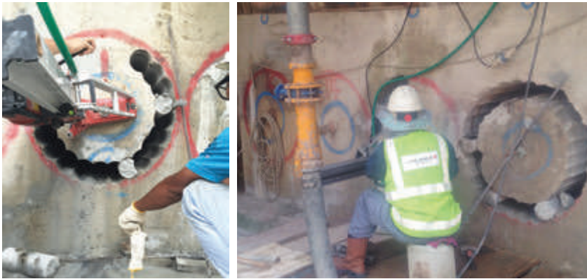
Figure 4: 24 cores to complete stitch coring of secant bored pile
