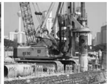
Figure 11b: Secant bored piles wall installation and reinforcement of ‘male’ piles
