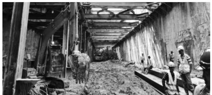
Figure 9: Bottom up excavation in Kenny Hill formation at the Merdeka Station
