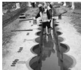
Figure 11a: SBP guide wall being prepared prior to drilling works
