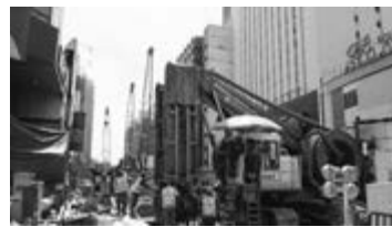
Figure 6: Low Headroom 'Hydrofraise' D-wall machine at Bukit Bintang Station
