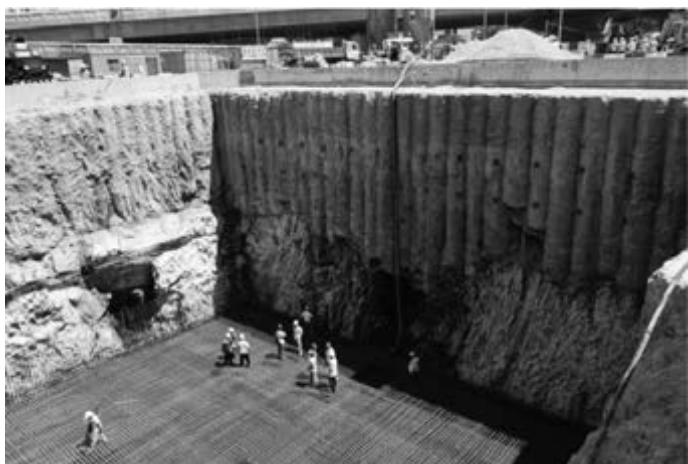
Figure 3: Deep Soil Mixing Wall on undulating rockhead
