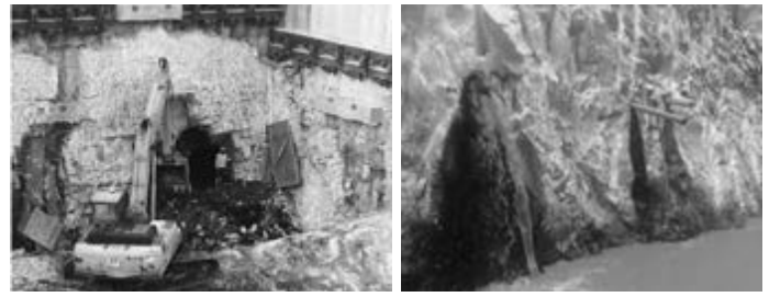
Figure 25: Photos showing sizes of cavity affecting TBM operation
