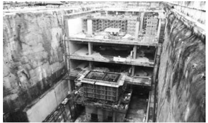
Figure 20: Partially completed Cochrane Station Box
