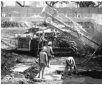
Figure 12: Installation of Temporary Ground Anchors for the SBP wall
