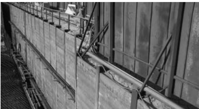
Figure 2: Soldier pile timber lagging with well point dewatering
