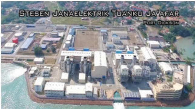
The Tuanku Ja'afar Power Station in Port Dickson
