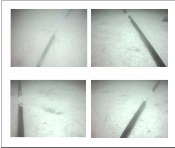
Fig.6 Typical examples of occluded pipeline
