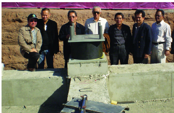
Figure 2: The first bearing for the Iranian project installed on 9 November 2007
