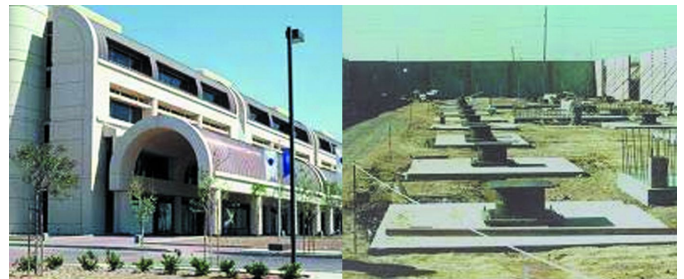
Figure 1: (Left) San Bernardino County Law and Justice Centre. (Right) Rubber bearings installed on foundations
