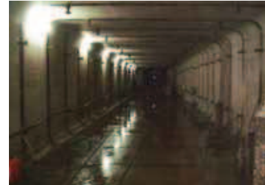
Completed sections – accurately done
