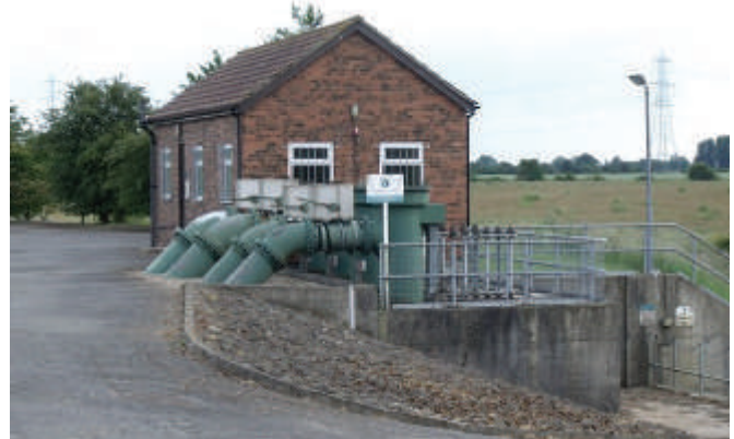
Photo 7: A Typical Pumping Station
